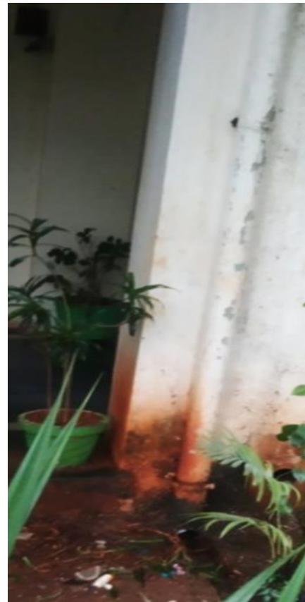
RO Waste water pipe line
